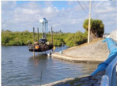
Here today gone tomorrow. This research barge was working at the West Lake Bridge on the the West side and then it moved to the East side collecting core samples under the water. Then it disappeared as quickly as it appeared. Core samples are for scheduled work in the future according to Jim Higgins.
